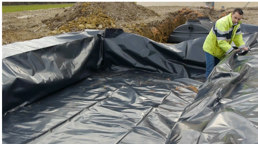
Figure 25 – Installation de la membrane souple
